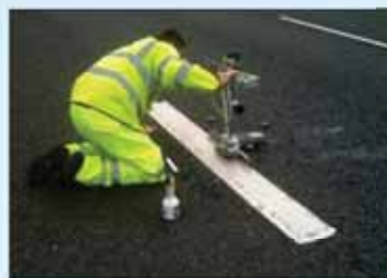
Road Marking Test
