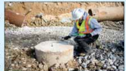
Pile Integrity Test
