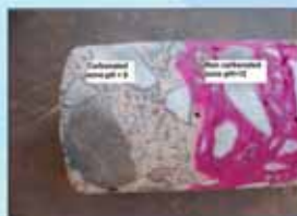
Carbonation of Concrete
